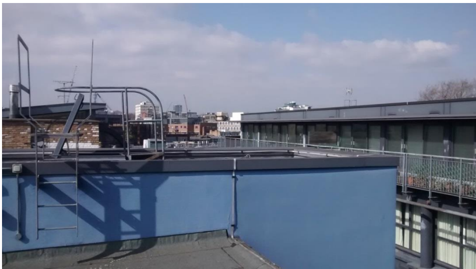
Image 2: Photograph from roof of Zinc House showing relationship to City Pavillion
